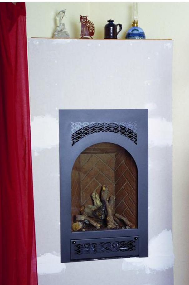
This attractive Avalon Hideaway fireplace by Travis Industries of Mukilteo, Washington, heats rooms of up to approximately 650 square feet in Seattle's marine climate. The Avalon Hideaway takes in fresh air from—and vents to—the outside of the house.
